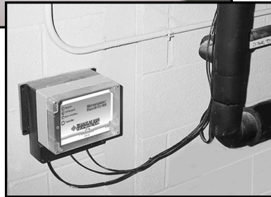
Solenoid wrapped pipe (Coil hidden by insulation) with deposit controller
