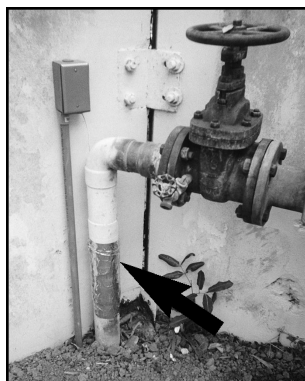
The coil is wrapped around a 2" water pipe and protected from dirt, disturbance and moisture with weatherproof tape.
