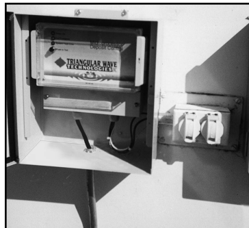
Triangularwave Technologies, Inc. Microprocessor TWT-5C8-402 installed in a weatherproof electrical box on the outside wall of the building.
